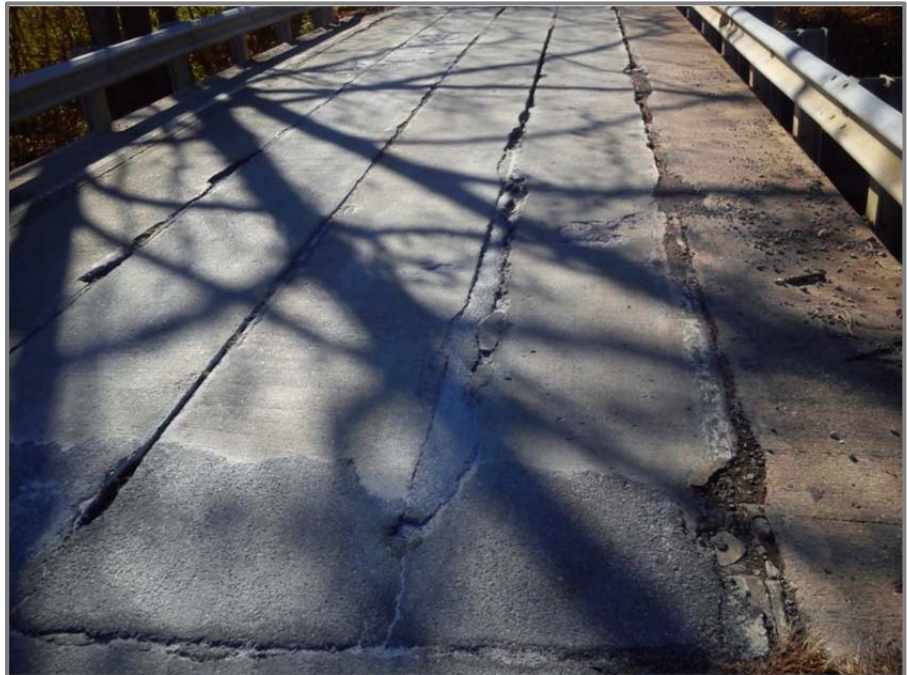
(Broad Run Road Bridge crossing Back Run Creek, leading to Floyds Fork)
